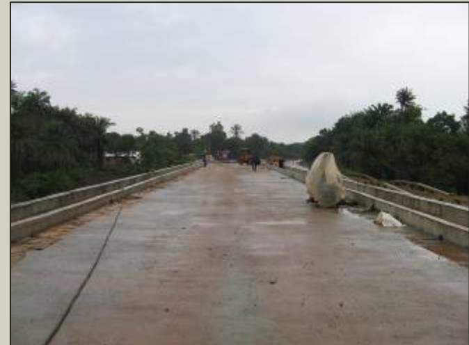
Boke Bridge almost completed
