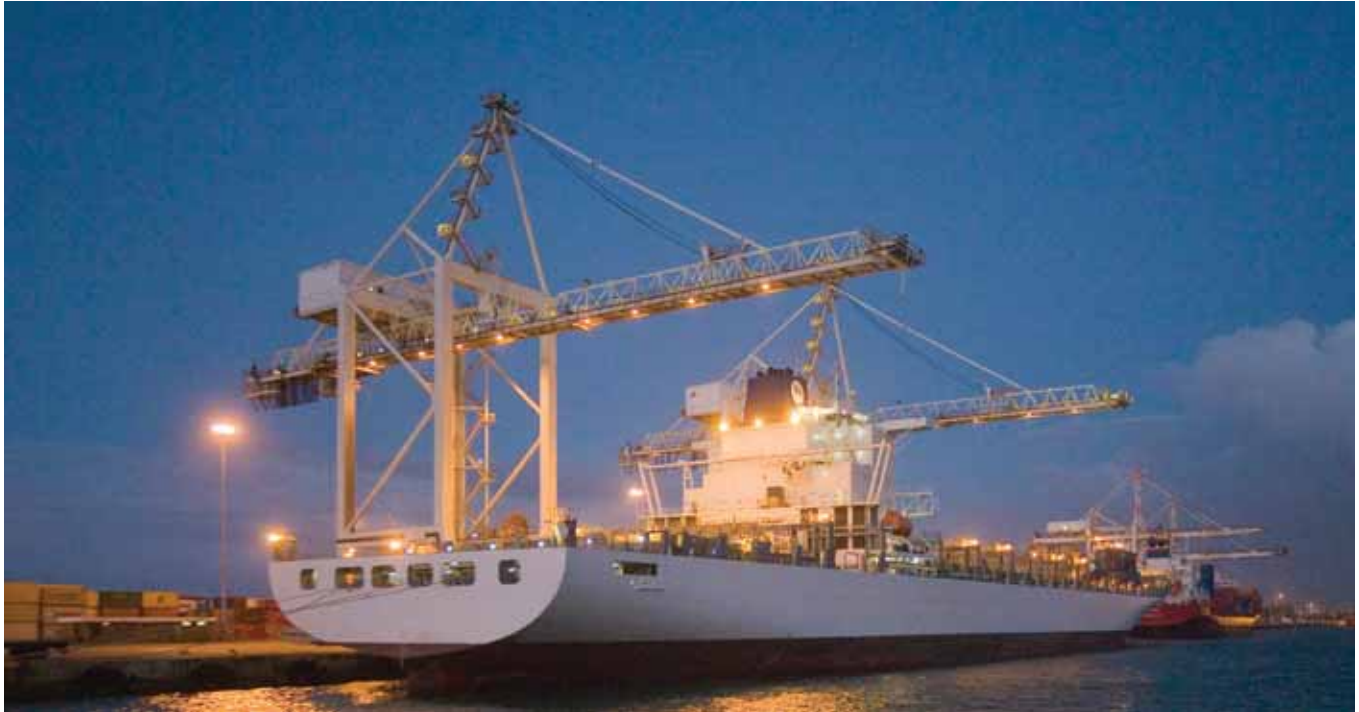
National Ports Authority plans to spend approximately R18,5 billion in the next five years upgrading infrastructure in the seven ports it manages
