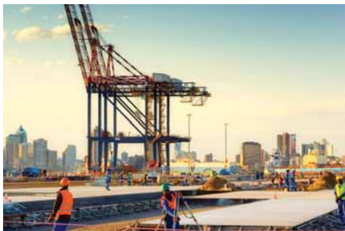
Construction work being performed at Durban's Pier 1 Container Terminal.
