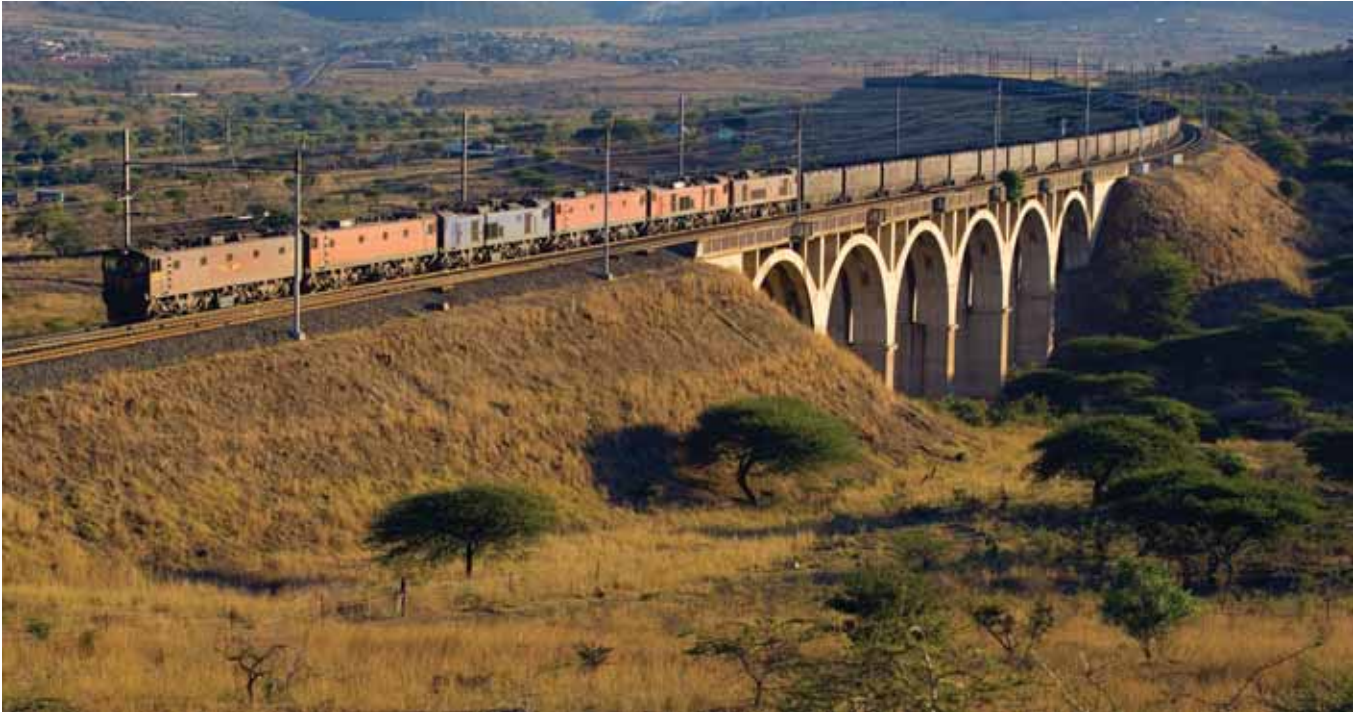
Freight Rail's infrastructure represents approximately 80% of Africa's rail network.
