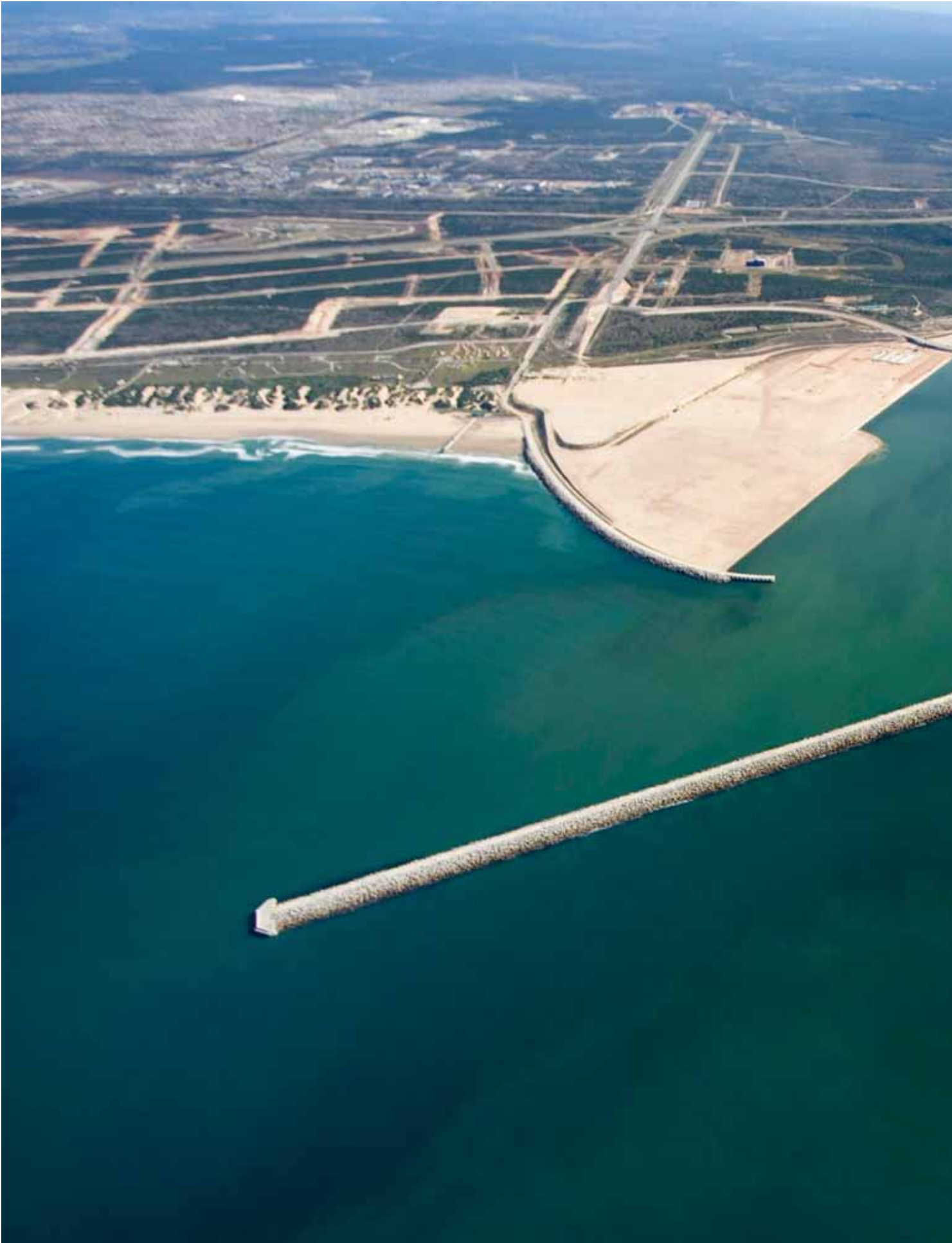
Construction of the new Ngqura Port, outside Port Elizabeth, with a two berth container terminal, is under way
