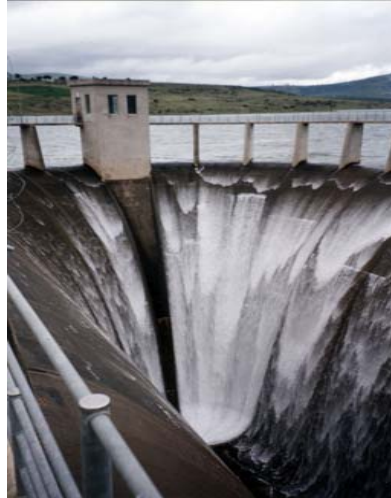
Binfield Dam Spillway
